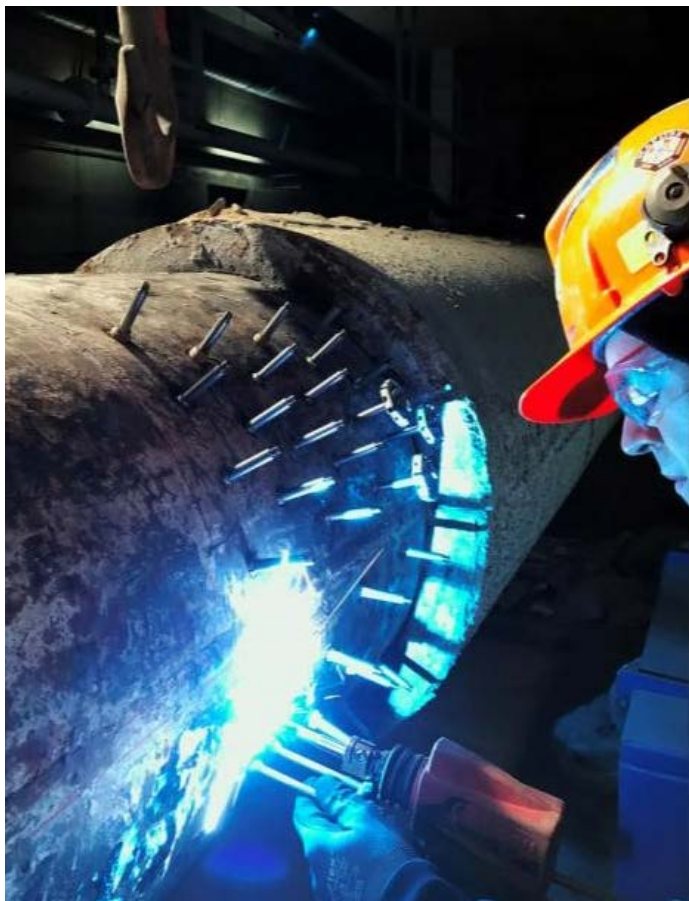
Figure 8. Rapid Arc Welding - Attaching a stud within 0.5 secs
